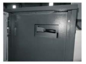
Remove the boiler side panel.
